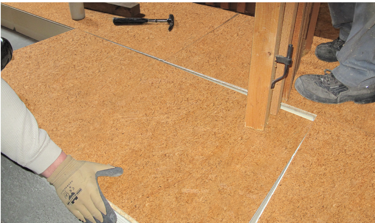
LINITHERM attic insulation PAL or PGV LINITHERM PE vapour barrier 120 Wooden beam ceiling Rafter
