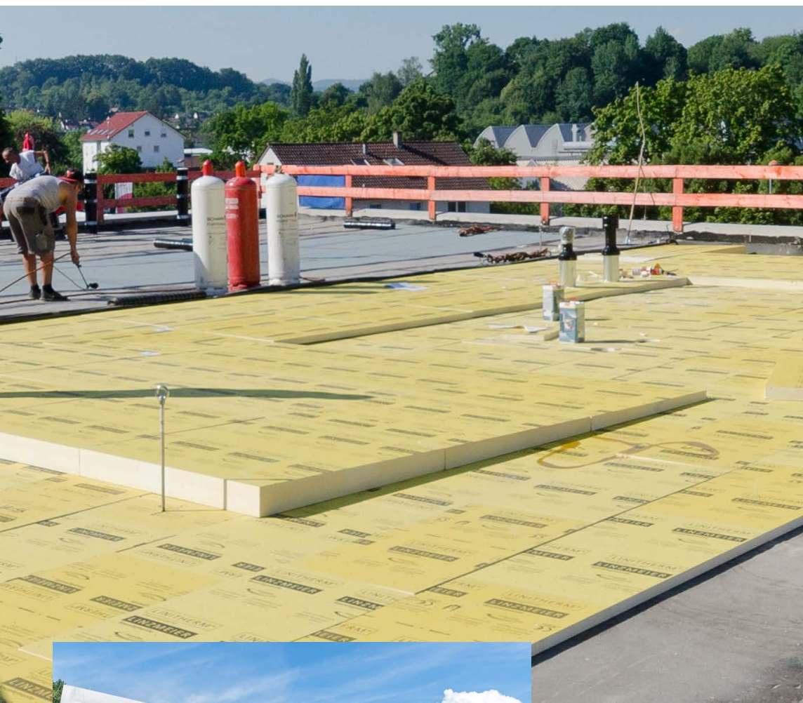
LINITHERM PGV gradient insulation Wannweil fire station
